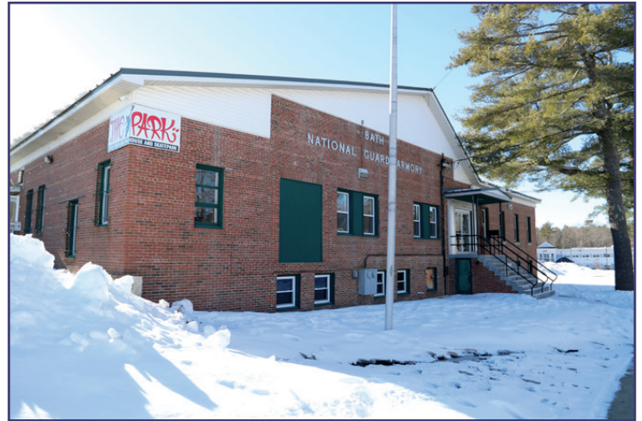
The Bath Youth Meetinghouse & Skatepark is located in the former National Guard Armory, which was built in 1938 and dedicated in 1939
