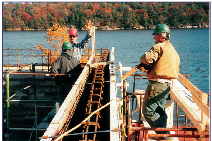
Photos from the construction of the current wastewater processing facility, circa 1991, courtesy of the Bath Water Pollution Control Facility
